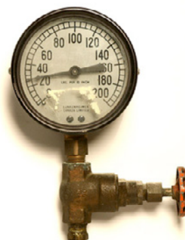
→ Pressure gauge from the Youville Pumping / PAC 1998.5 © www.lucbouvette.com
